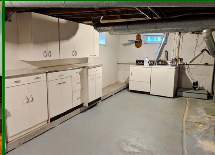
Laundry in Basement
